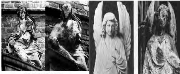
How acid rain affects stonework. The picture on the left was taken in 1908
